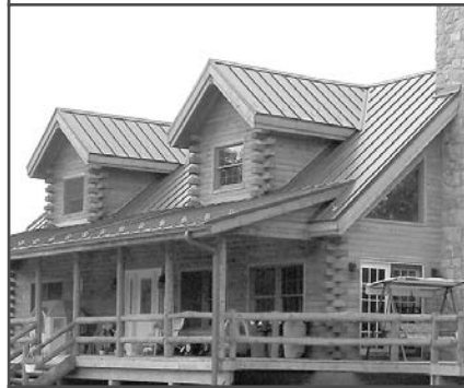
If you saw a metal roof 20 years ago, it probably looked like this. It’s called a “standing-seam” metal roof and consists of vertical panels arranged side by side and fastened at the seam.
