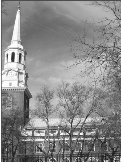
Located a few blocks down Market Street from Benjamin Franklin's print shop in Philadelphia, Christ Church was built between 1727 and 1747 and features a standing-seam copper roof.
